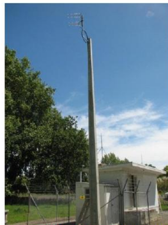
Figures 9 and 10: Photographs of the BRU and LRU Installed on the UNL Pole and the RRU Antenna at the Eskdale Zone Substation Respectively
