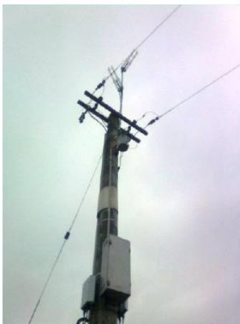
Figures 9 and 10: Photographs of the BRU and LRU Installed on the UNL Pole and the RRU Antenna at the Eskdale Zone Substation Respectively
